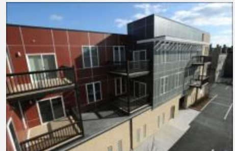
King Drive Commons IV - continues progress started by Commons I
