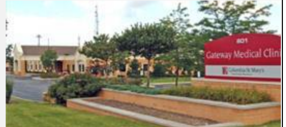
Gateway Medical Clinic – boosting health services in an area that ranks as only 60 percent the area median income.
