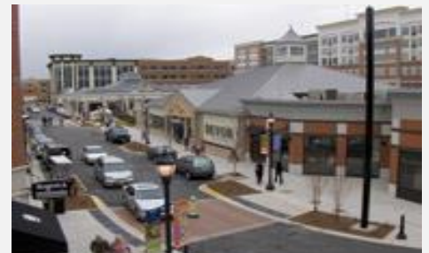
Former dump site becomes regional mixed use center
